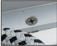
Stainless steel screw aluminium floor rail
